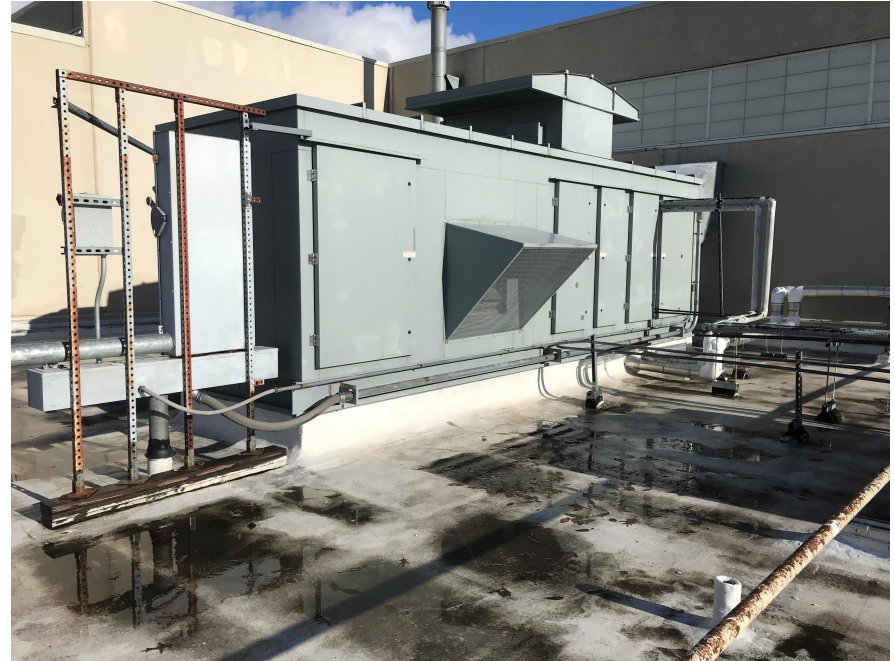
Dektron Unit Replacement: Pool Dehumidification
