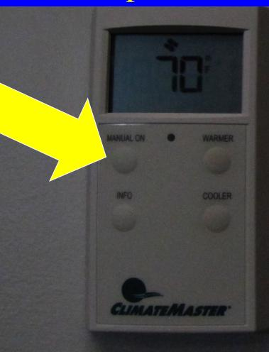
After school hours, press Manual On only ONCE to reset to daytime temperature; repeat as needed each time temperature sets back (about an hour later)
